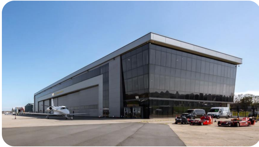
6000 SQ M, BUILDING 510 IN LONDON, UK
